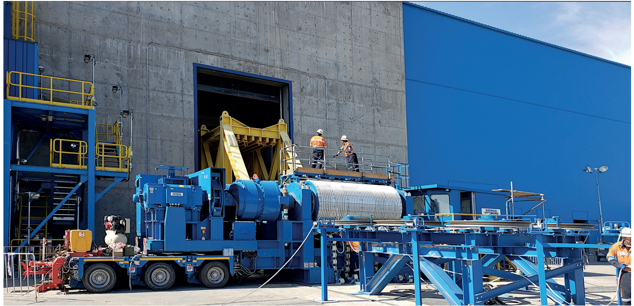
Preparations for rope laying: the mobile friction winder in front of the machine house, in the foreground the horizontal deflector sheaves.
