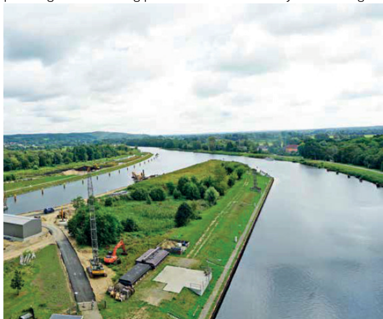
Last exterior works around the new building (© Alexander Rechenbach)
