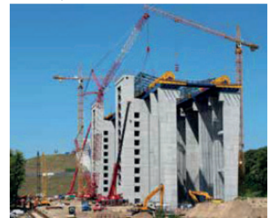
Installation of an element of the rope pulley hall (both © WNA)
