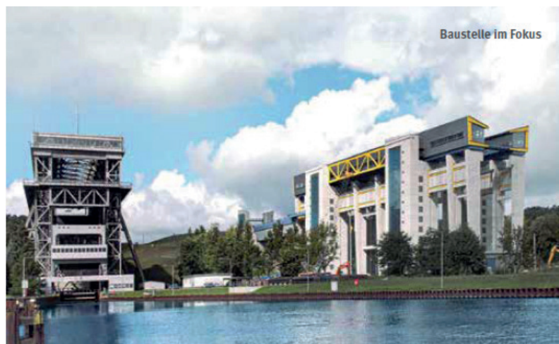
Old structure side by side with the new structure in September 2020. Both will operate together for about five years. (© Bärbel Rechenbach)
