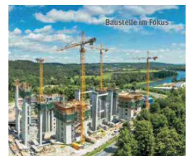
Assembly of reinforced concrete structures
