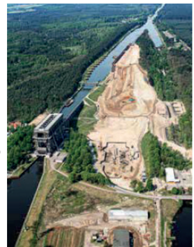
Construction of the building pit next to the historical hoist (© WNA)
