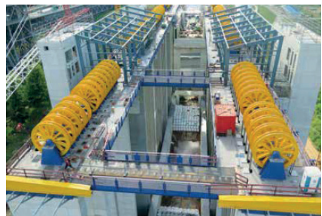
View into the axis of the ship lift (© WNA)
